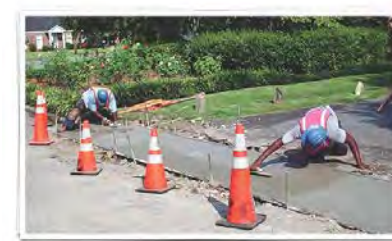
CITY CREWS INSTALLING SIDEWALKS
