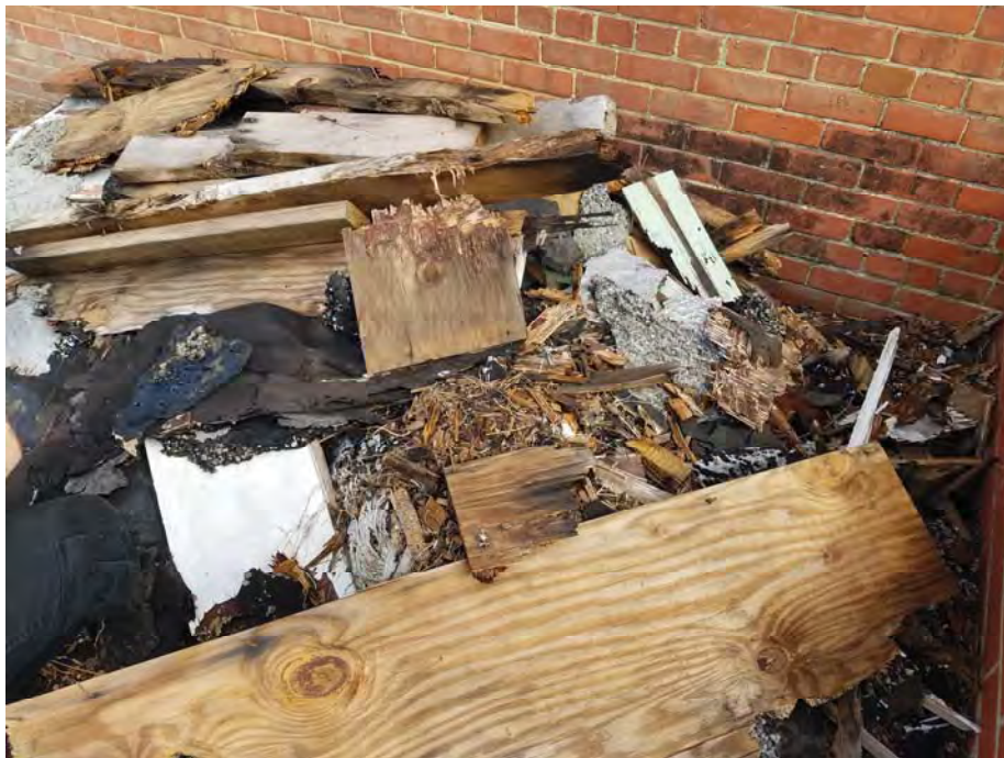
Example of asbestos-containing roof debris outside Building 2
