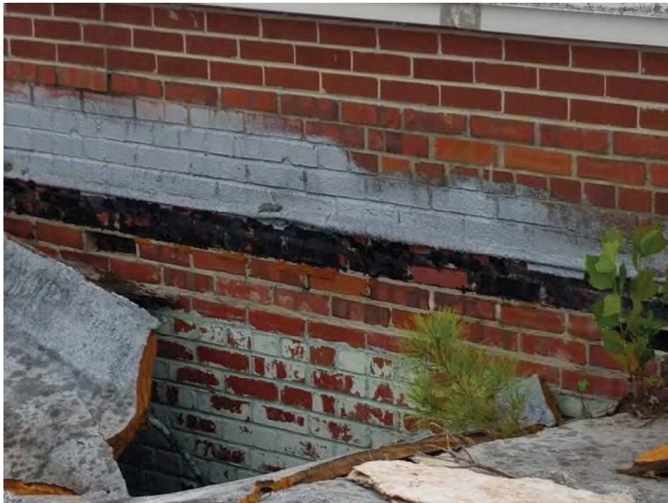
Example of roof flashing on Building 3
