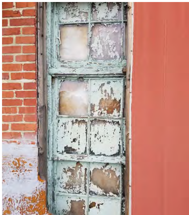
Example of window glazing on roof of Building 3
