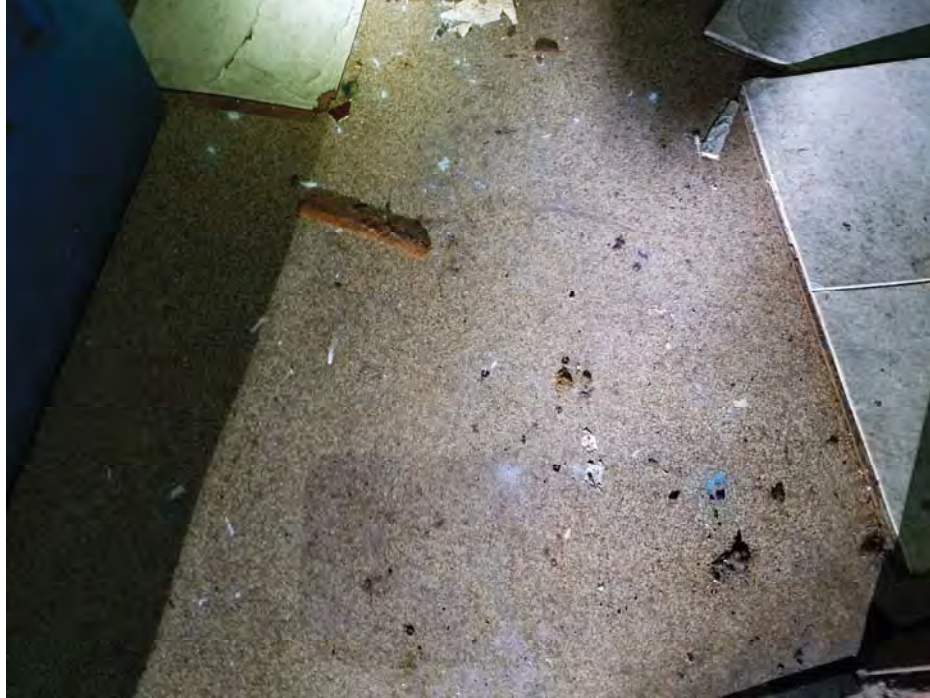
Example of tan vinyl sheet flooring in Building 3
