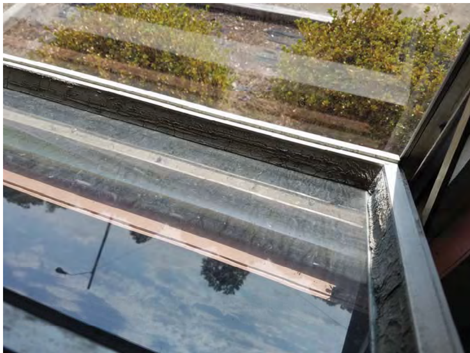
Example of window glazing on metal windows in Building 2
