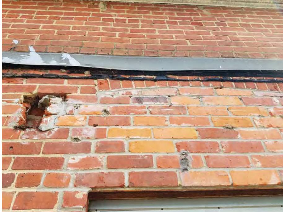
Example of stoop mastic on Building 2
