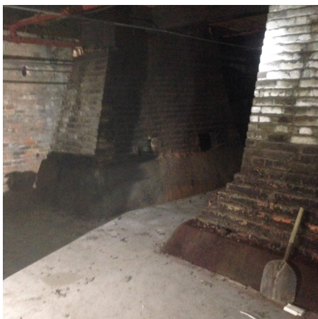
Photo 9 – View of coal furnaces located in the basement of the former mill
