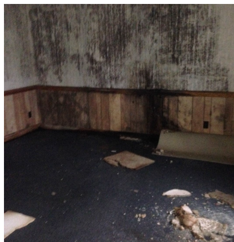
Photo 12 – Wall staining observed in the former mill
