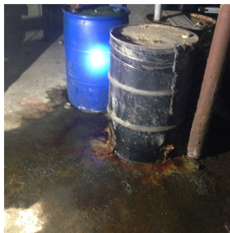
Photo 8 – Stained concrete and leaky drum inside former mill (basement)
